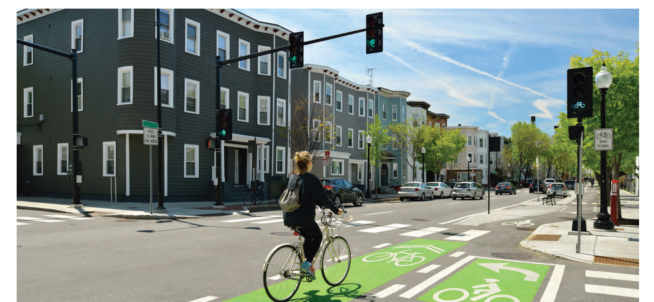
On-Street Bicycle Lane Through an Intersection
