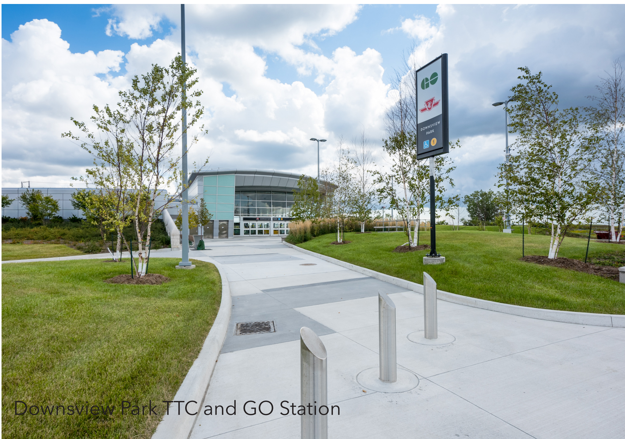
Replacing the pedestrian bridge with a new pedestrian gateway with connection to Downsview Park to come
